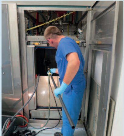
Figure 13a: On-site rehabilitation of an interior surface on a chamber using electrochemical (anodic) cleaning (source: Henkel Beiz- und Elektropoliertechnik)
